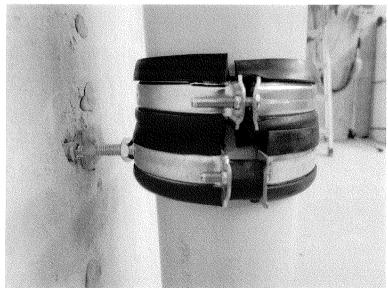
Mounting of the clamps for the wastewater system "SILENTA FR (FLAME RETERDANT) ATIKSU BORUSU 110 x 5.3" (manufacturer: GF Hakan Plastik) with acoustic pipe clamps (double clamps, supporting and fixing clamps) "GF Hakan PLASTIK 110-119, 116-125" (made by GF Hakan Plastik). To avoid contact between supporting (loose) clamps and the pipe, 2 spacers (2 x 7.5mm) on each side of the clamps were used. Mounting details see figure 1.
